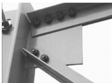
Figure 7-17. Misc. Connection: Truss Column C2 / Truss B7
